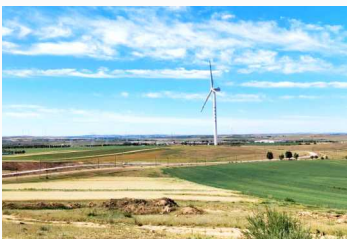
Kangbao Wind Farm in Zhangjiakou, Hebei
