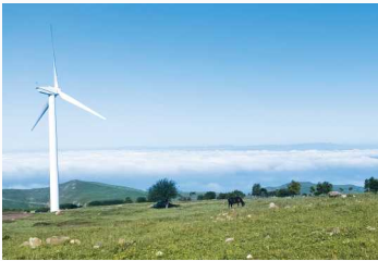
Aerial Grassland Wind Farm in Wei county, Zhangjiakou, Hebei Province
