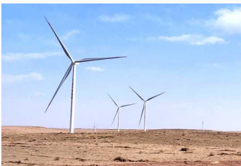
Taiyangshan Wind Farm in Wuzhong, Ningxia
